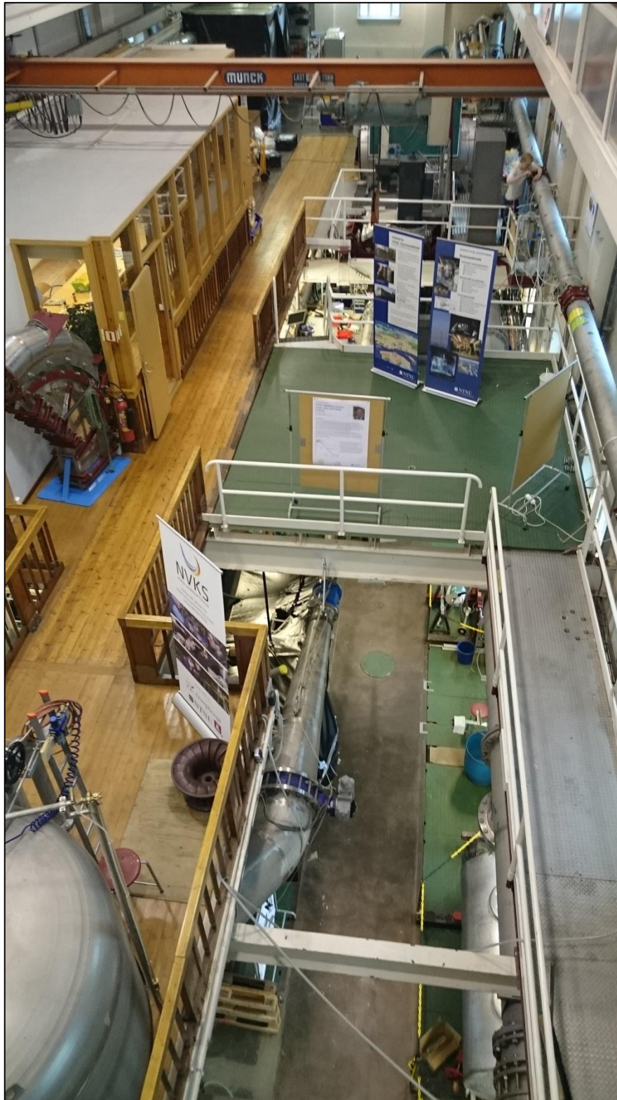
Figure 8: Picture of the first floor. Picture taken from northwest.
