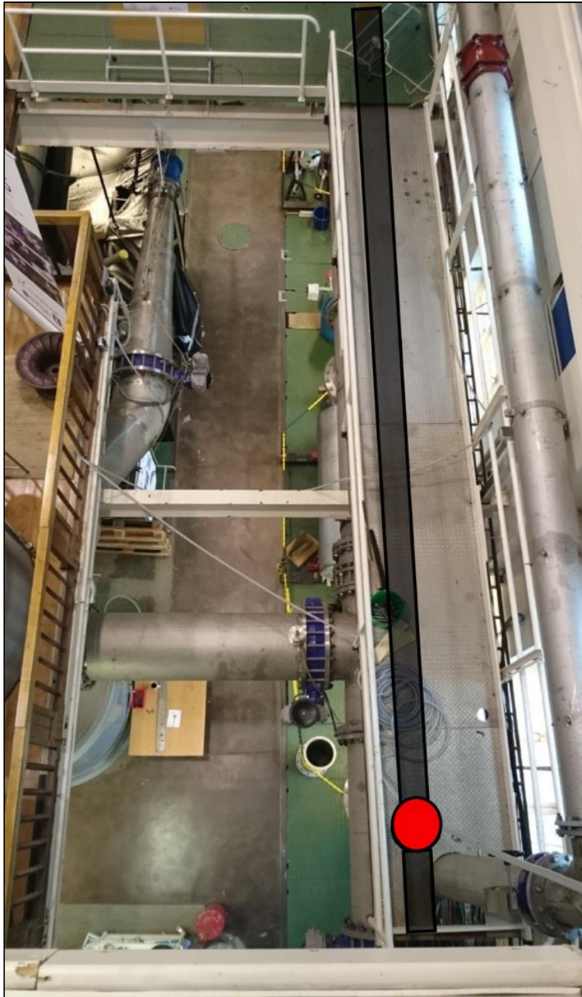
Figure 17: Suggested location of the surge shaft.
