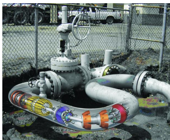
Figure 13 Corrosion control by scraping and pigging (O'Meara, 2006)
