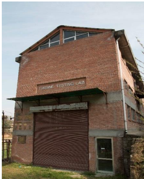
Figure 3.7: Turbine Testing Laboratory
