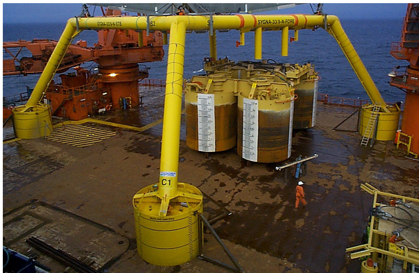
Picture 23: This picture gives a good impression on how massive subsea structures can be
