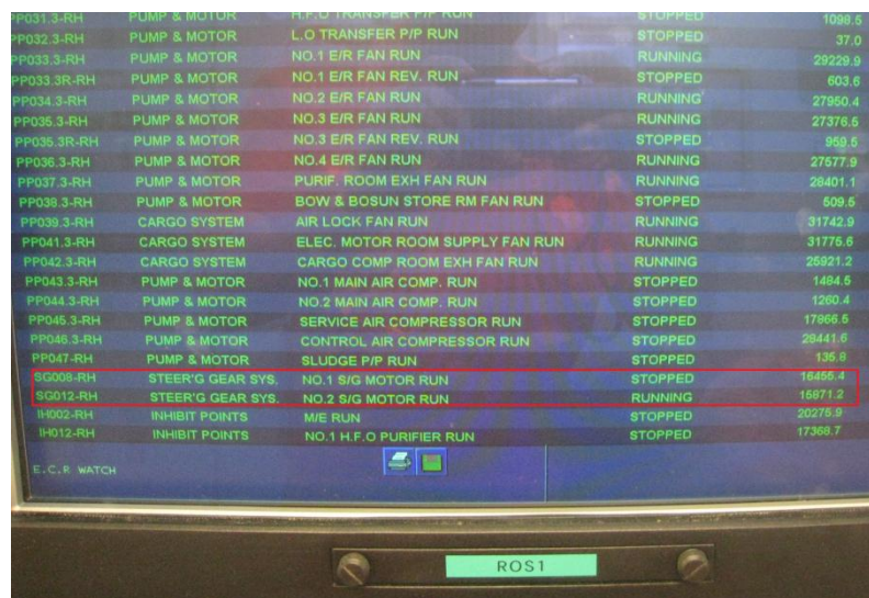
FIGURE 25: STEERING GEAR PUMPS IN ROS
