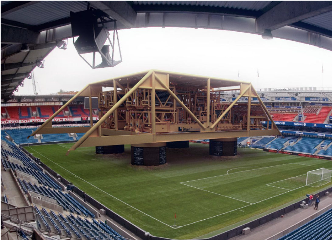
Figure 2.5: The SCSt placed in a football stadium (Ullevaal) [64]
