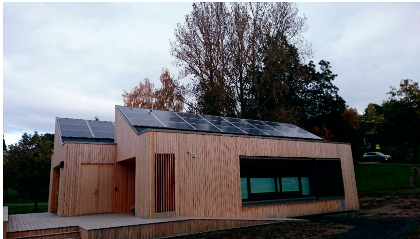
Figure 42. The ZEB Living Lab, as seen from the south. (Photo: Clara Good)
