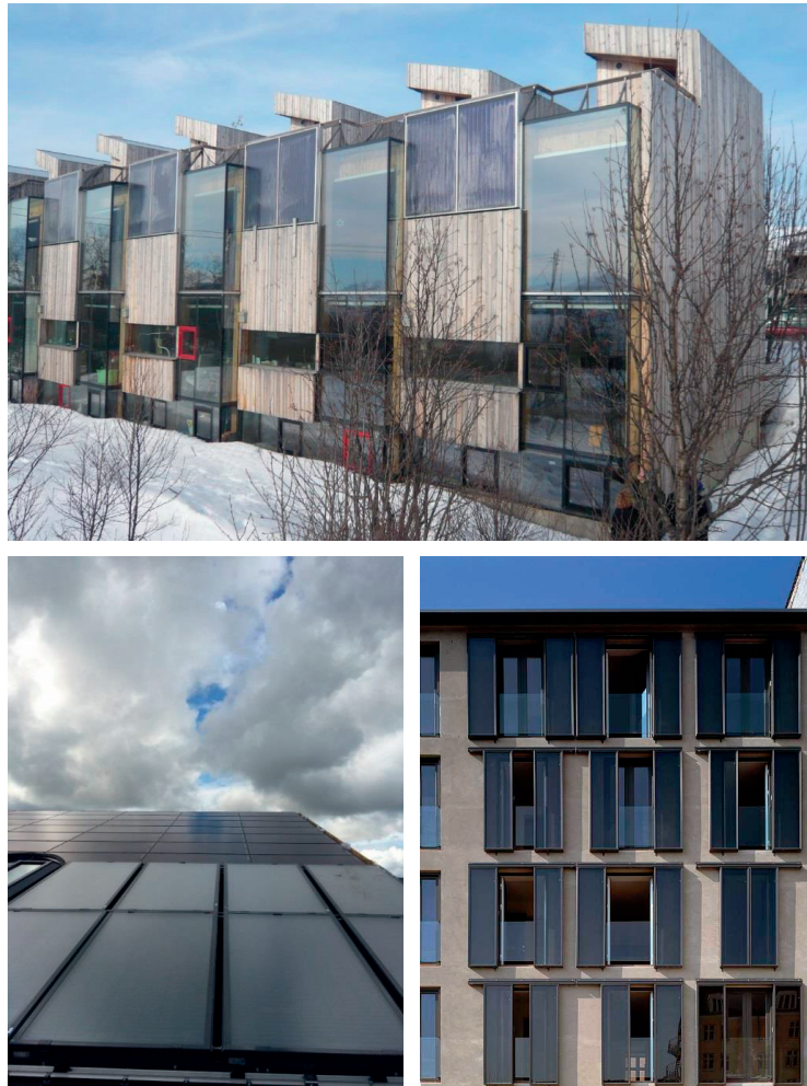
Figure 8. Different approaches to building integration of solar thermal systems. Clockwise from top: Façade integrated flat plate solar collectors in Storelva passive houses in Tromsø, Northern Norway (photo: Solvår Wågø, NTNU/SINTEF Byggforsk), solar thermal collectors used as solar shutters in Copenhagen (photo: CF Møller Architects), roof-added solar thermal collectors at Multikomforthus, Larvik (photo: Harald Amundsen, Brødrene Dahl).
