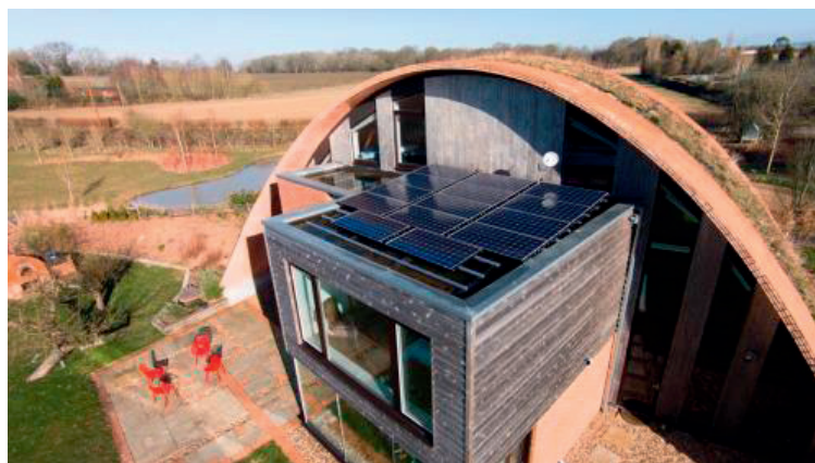
Figure 22. The Crossway passive house, using flat plate PV/T modules from Solimpeks. Photo: Hawkes Architecture.
