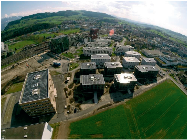
Figure 25. The Suurstoffi PV/T installation from above. Photo: Simon Büttgenbach/Meyer Burger Group.
