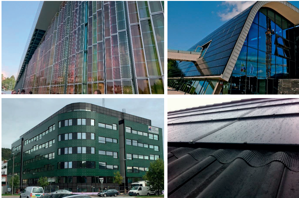
Figure 9. Different approaches to building integration of PV systems. Clockwise from top left: the Grätzel cell façade at EPFL in Lausanne (photo: Clara Good), building integrated PV modules at Oseana kunst- og kultursenter in Os (photo: Tove Heggø/Creative Commons), roof integrated PV at Skarpnes zero energy neighbourhood in Arendal (photo: Hans Kristian Sonesen, Skanska), and green façade integrated PV modules on Solsmaragden in Drammen (photo: FUSen AS).
