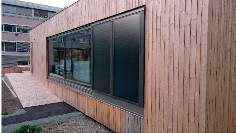
Figure 44. The façade-integrated solar thermal collectors on Living Lab. Photo: Clara Good.
