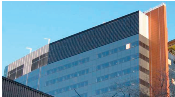
Figure 18. The SolarWall PV/T facade at Concordia University, Montreal. The PV/T system is the dark blue area on the upper part of the façade. Photo courtesy of Conserval Engineering.
