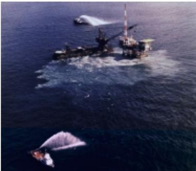
Figure 2.1: Picture of a blowout resulting from SCP (Bourgoyne et al. 1999).
