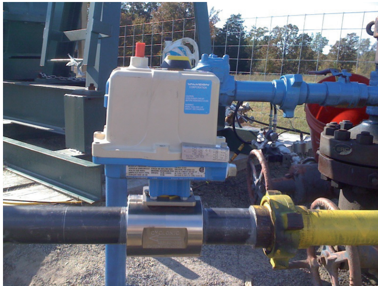
Fig. 1.16 – The remotely controlled choke installed on the Noblin #2. A motorized actuator (gray and blue box) is mounted on top of the choke. The actuator receives a control signal from the RTU to open or close.
