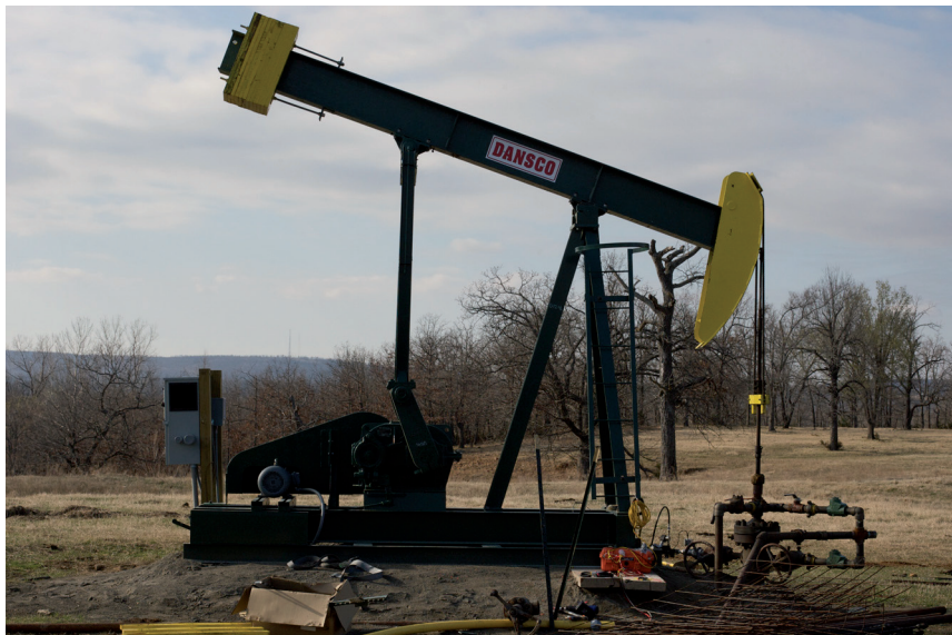
Fig. 1.17 – The pumping unit installed on the Noblin #2.
