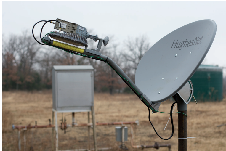
Fig. 1.20 – The satellite dish installed on the Noblin #2.
