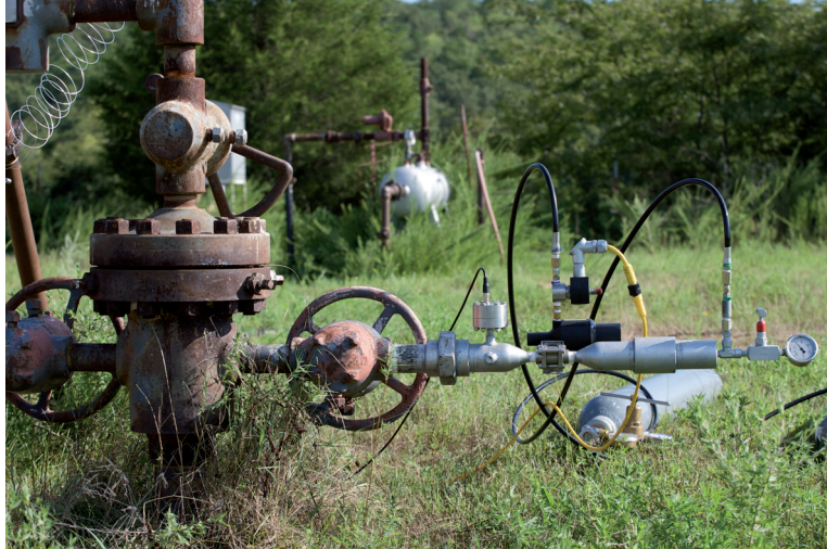
Fig. 1.5 – The Acoustic Fluid Logger IV gun mounted on a well. The nitrogen tank pressurizing the gun can be seen in the background.
