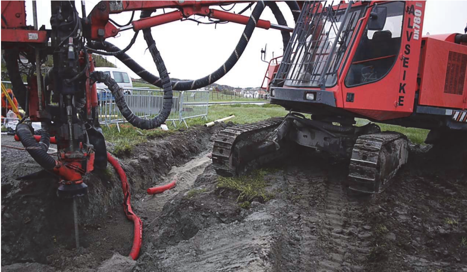
Figure 3.8: Drill rig used for installation of vertical soil temperature sensors.
