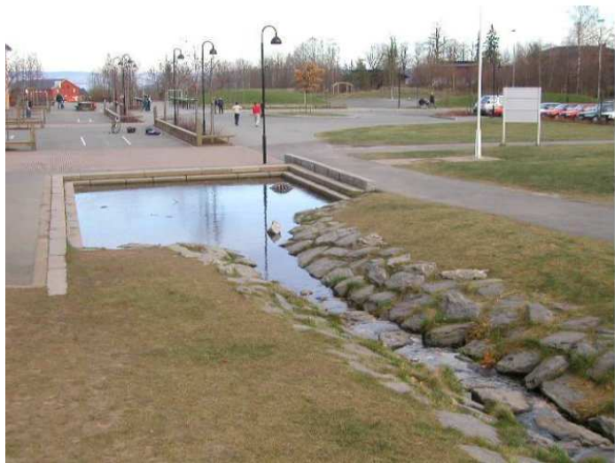
Figure 17: Example swale design. Source: (kommune, 2014)
