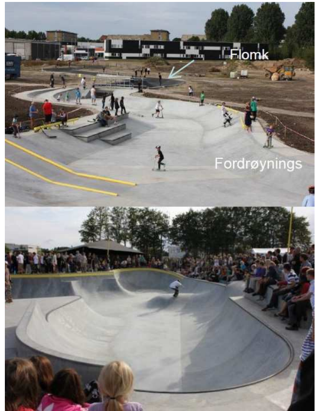
Figure 19: Example of dry basin in Roskilde, Denmark. Source: (kommune, 2014)
