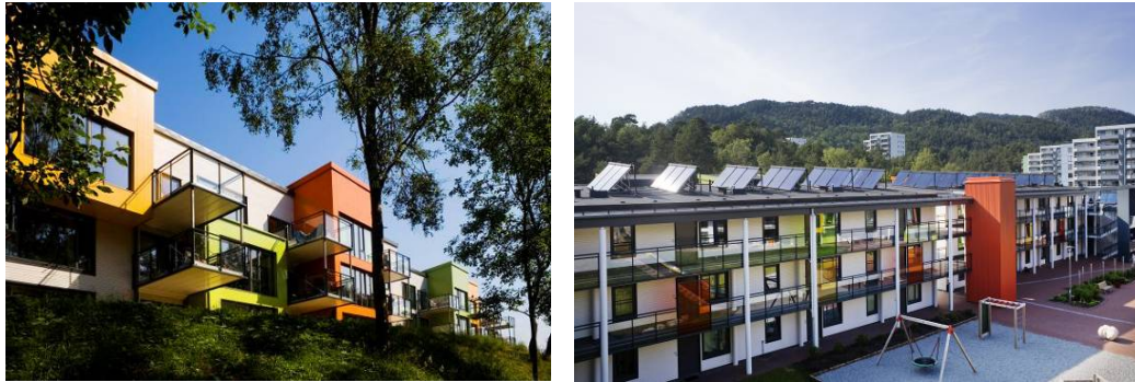
Fig. 3 and 4: The passive house with balconies, oriels and living rooms facing west (left picture) and entrances to the common outdoor space. (right picture) Solar collectors on the roofs facing south. Photo: Knut Egil Wang
