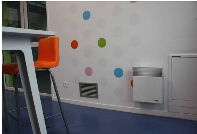
Figure: There is no central heating in the kitchenette, but a little radiator. The ventilation is mechanical and the heat produced is not recovered.
