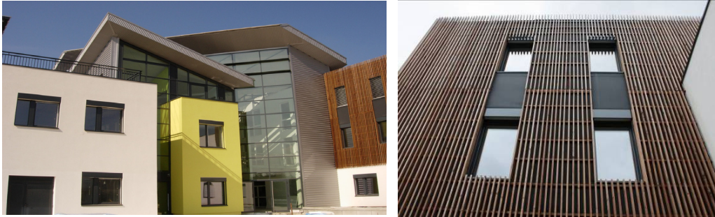
Figure: Vertical timber cladding in combination with glazing and sanded surfaces.
