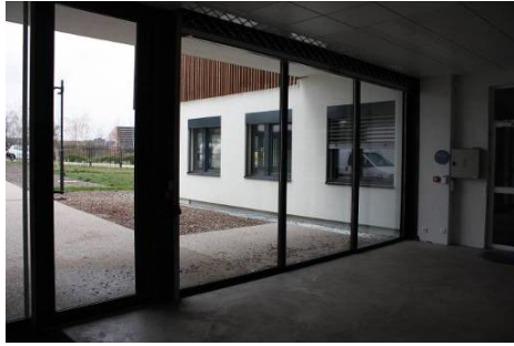
Figures: Natural ventilation of the atrium in summer: sliding doors at entrance level are open during the night (there is a security feature). The air goes through the skylight and refreshes the atrium.
