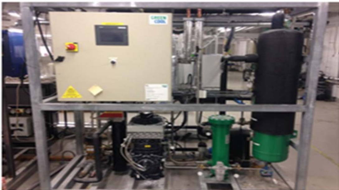
Figure 12 the second glycol cooler
