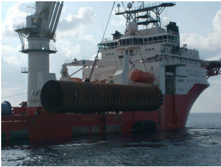
Fig: Lowering of a suction anchor
