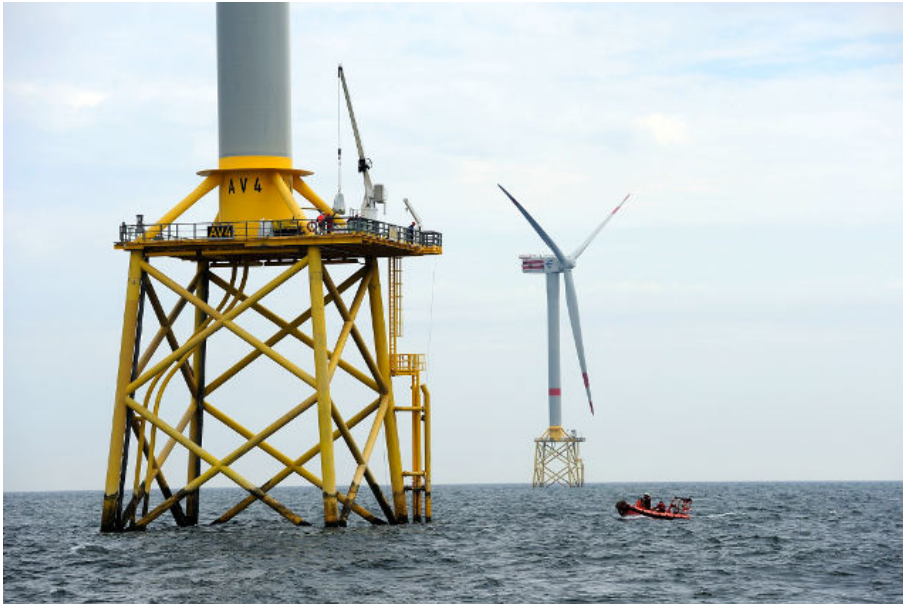
Figure 1.1: Jacket support structures in the Alpha Ventus offshore wind farm [3]
