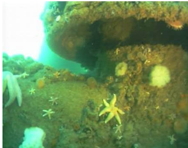
Figure 1.3: Snapshot of a boat-landing flange by an remote operating vehicle [4]
