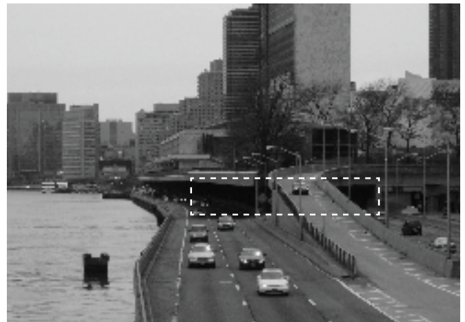
FDR view from North access
