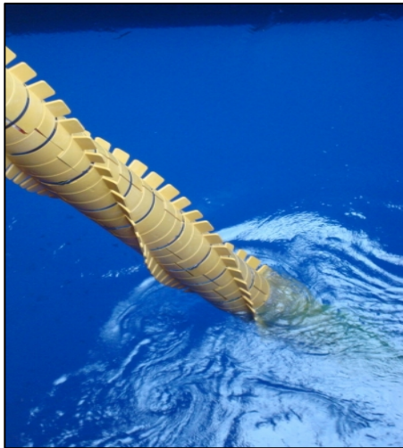
Figure 3-2: VIV strakes (Offshore-mag, 2011)
