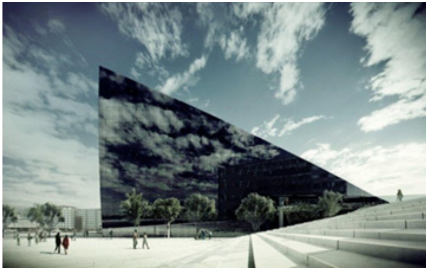
Figure 1. Illustration of the Powerhouse 1 building with its huge sloped roof integrated with PVs. Illustration: Snøhetta
