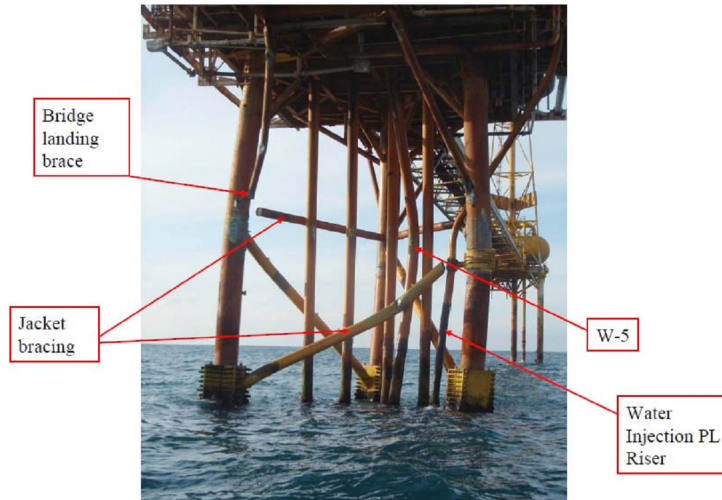
Figure 2.3: Ekofisk 2/4-W platform after impact.
