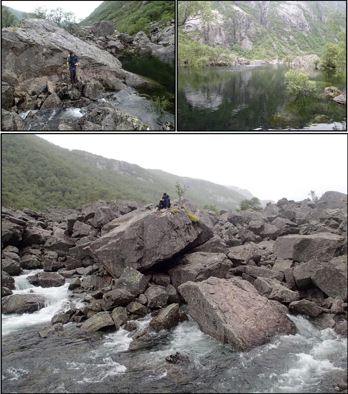
Figure 4.20: Upper left: Picture of the overflowing channel. The picture is taken close to point 4(Figure 4.18). Upper right: Picture of lake level response to intense rainstorm. Lower: Picture illustrating outlet of drainage through the dam, the picture is taken between point 2 and 3 towards northeast (Figure 4.18).
