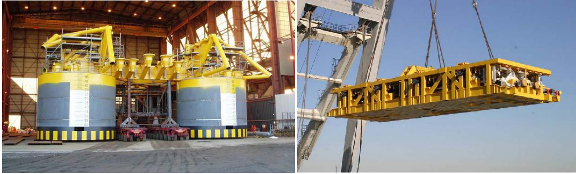
Figure 5: The foundation bottom structure to the left and the manifold module to the right [19].
