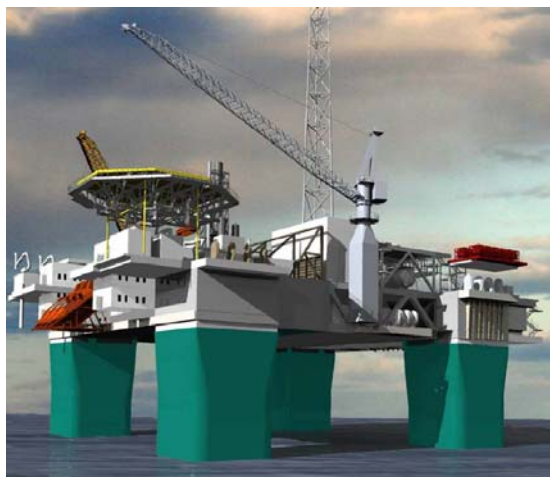
Figure 1. 1: General arrangement of Gjøa platform
