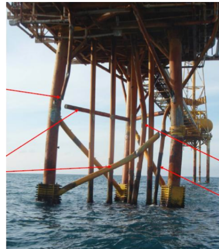
Figure 2.2: Undamaged and damaged north face of Ekofisk 2/4W
