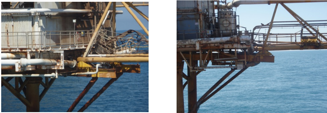
Figure 2.4: Bridge landing. Left: south. Right: north
