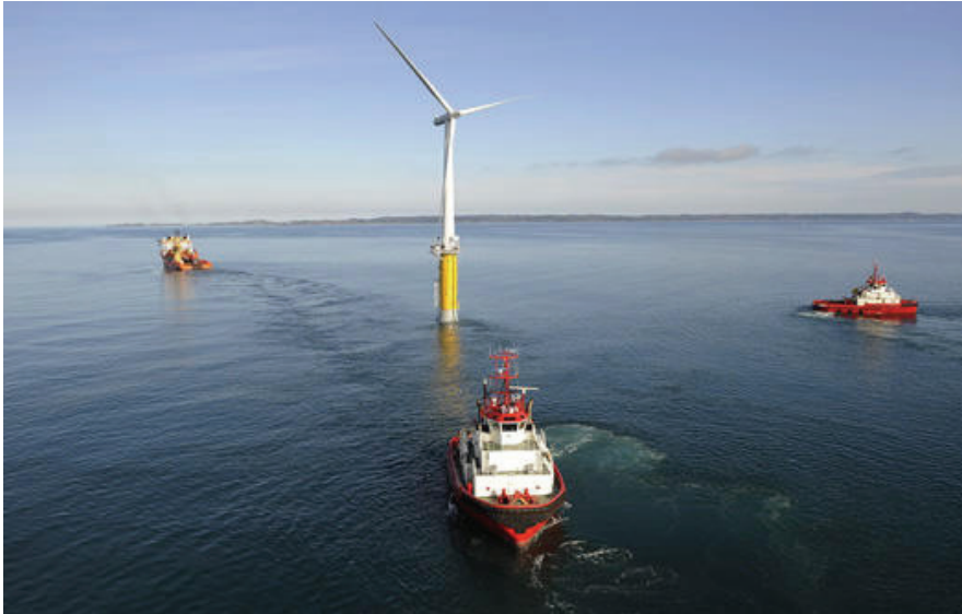
Figure 1.4: Hywind concept, 2.3 MW floating wind turbine (courtesy of Statoil).
