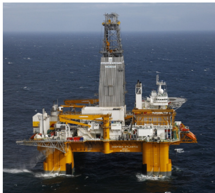
Figure 3-3: Deepsea Atlantic (Odfjell Drilling, 2009)
