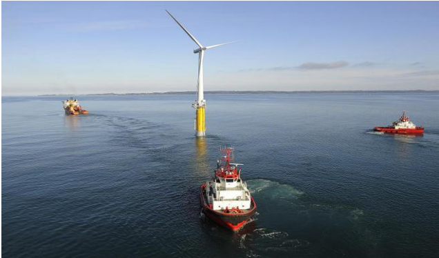
Figure 2 Towing of Hywind Demo (Statoil AS)
