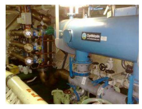
Figure 18: OptiMarin Installed on MV KCL Banshee
