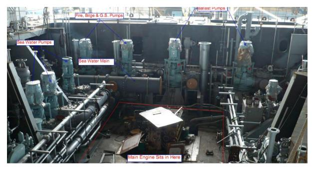
Figure 43: Tuju Arrow ballast pumps
