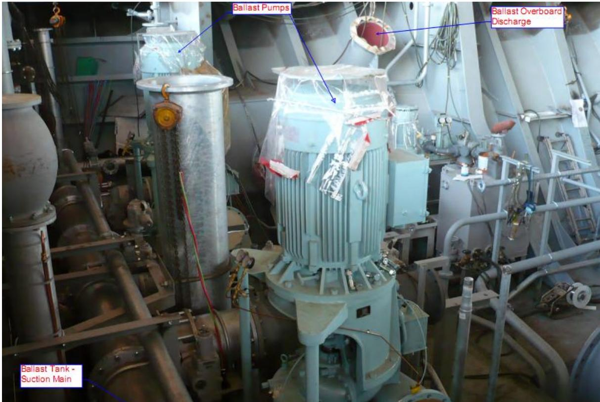
Figure 46: Ballast pumps and piping
