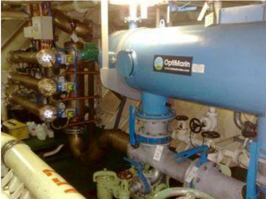
Figure 18: OptiMarin Installed on MV KCL Banshee
