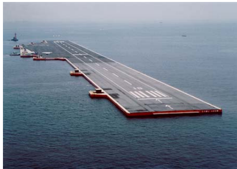
Figure 1.1.: MegaFloat, the largest floating runway prototype in the world, Tokyo, Japan is an example of a VLFS.
