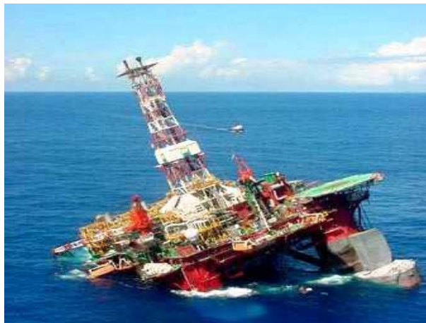
(c) Platform P-36: capsizing in damaged conditions.
