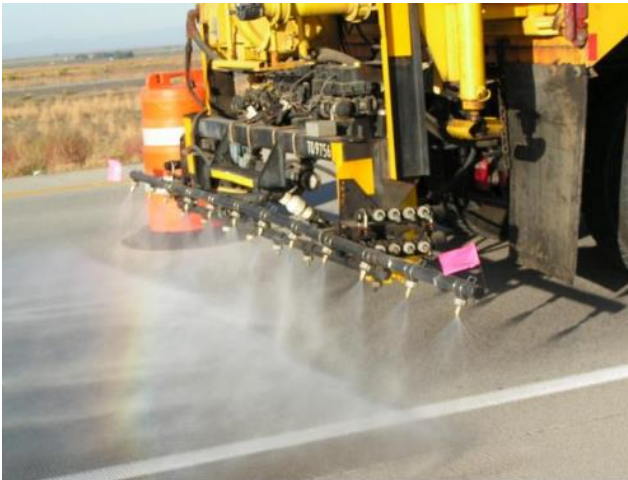
Figure 8.2 Photograph showing topical application of 30 percent-LiNO3 solution to concrete pavement.
