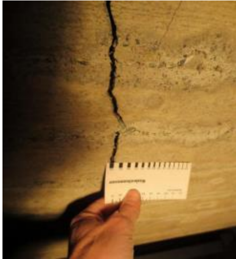
Figure 1. Crack (6 mm width) in internal beam of the bridge.
