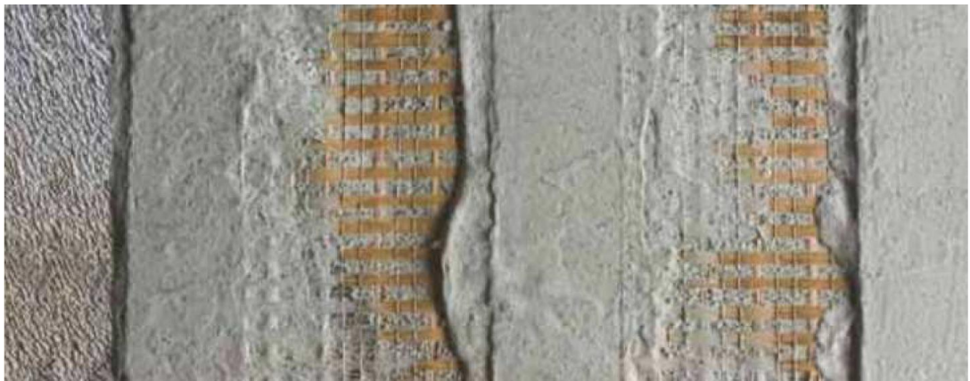
Figure 8.11 FRCM system with the PBO fiber on a cement matrix applied on the reinforced concrete element [70].
