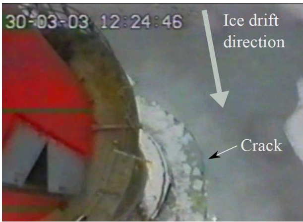
Figure 1.5 Semicircular crack approaching lighthouse.
