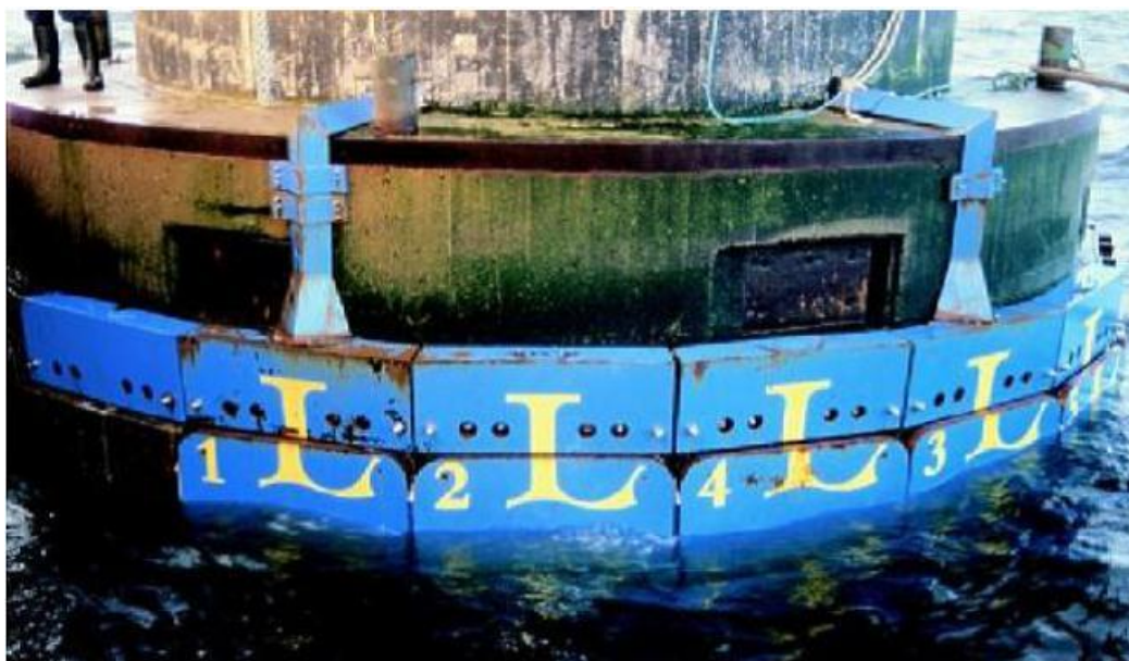
Figure 1.5 Force panels at Norströmsgrund (Bjerkås, 2014).
