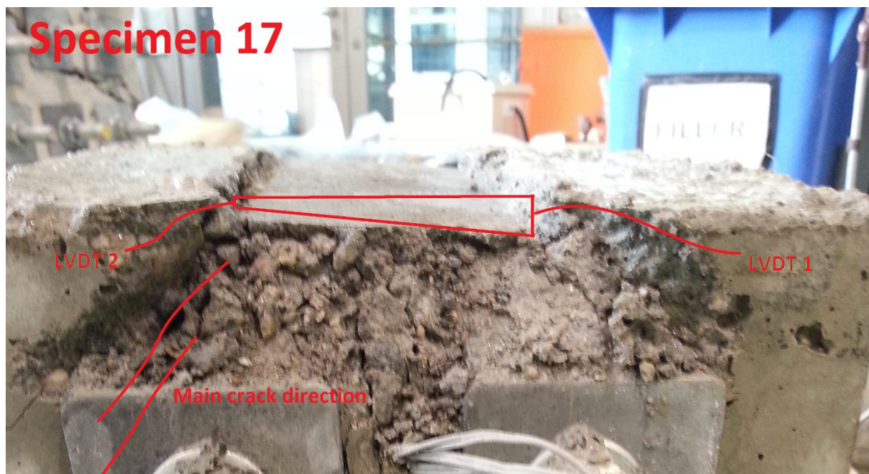
Figure 53 - Deformation under the loading area on specimen 17
