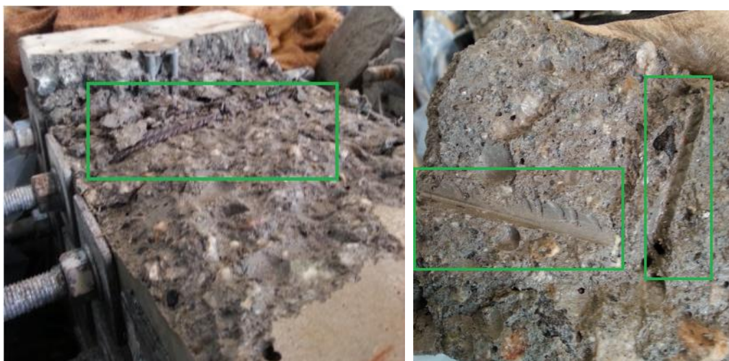
Figure 76 – Cracks appeared between steel and concrete
