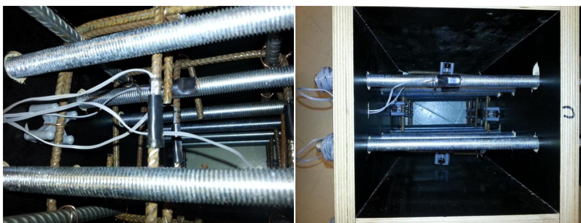
Figure 18 - Strain gauges mounted on reinforcement
