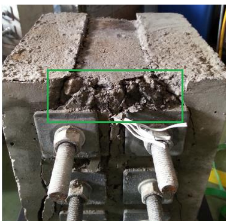
Figure 72 - Local crushing at the top
