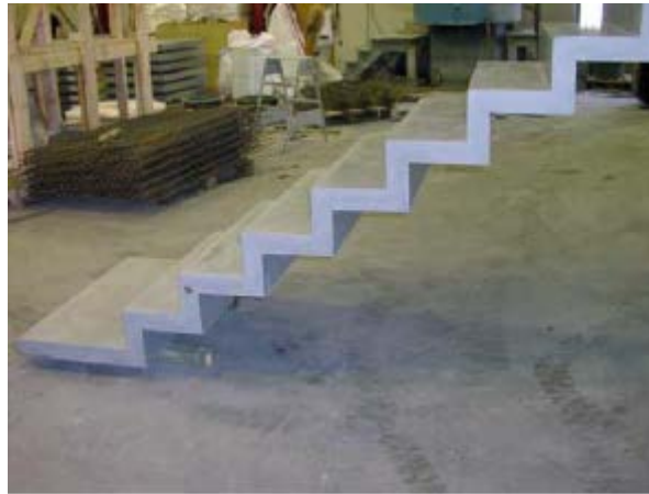
Figure 1-40 Example of staircase made of CRC. There are no supporting beams for the staircase; the load is carried by the steps
