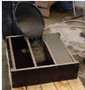
Figure 2-4 Pouring form bucket by short side
