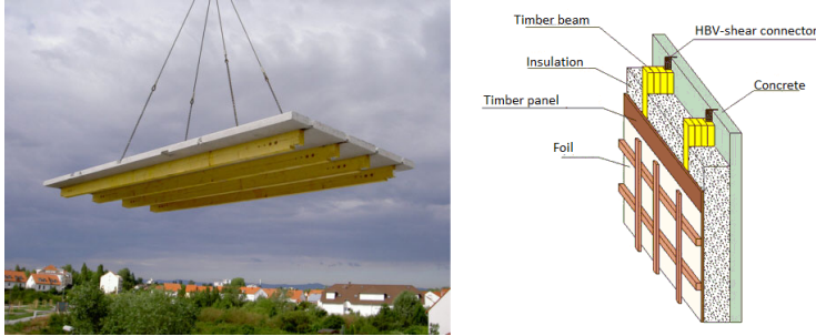
Figure 2.1: Example of an HBV-element and transportation on the construction site (from www.hbv-system.de )
