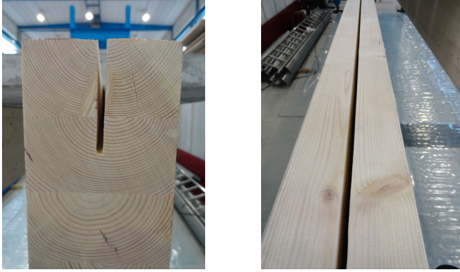
Figure 4.5: The slot routed in the glulam
