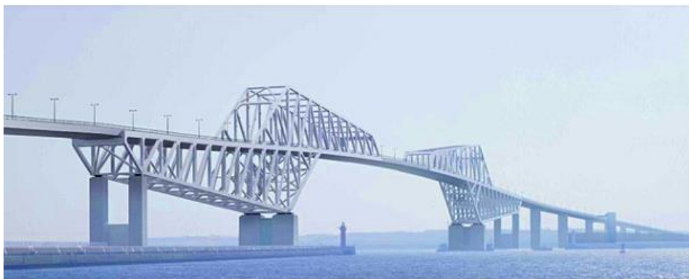
Figur 3.2: Tokyo Gate Bridge [18]
