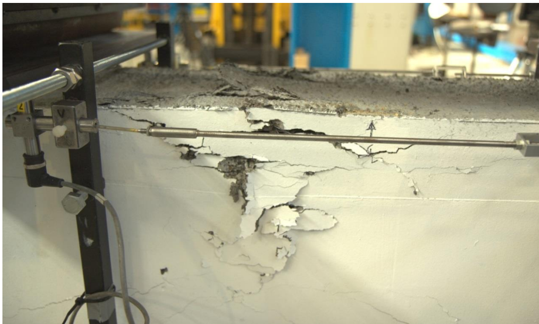
Figure 6.20. Final cracking on the east side of beam 2A.
