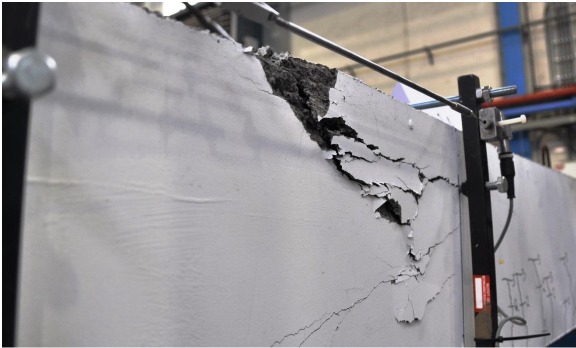
Figure 6.11. Final cracking on the west side of beam 1A.
