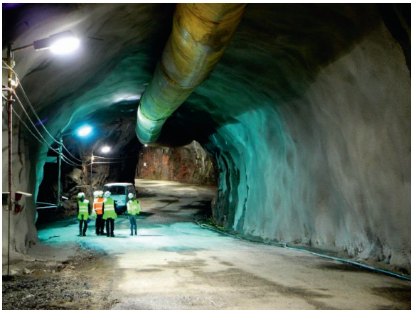
Fig. 24 The test section with SCL at Forsmark after completion.
