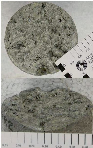
Fig. 8 Example of recordings of cracks in a sprayed concrete surface using a concrete crack measurement gauge
