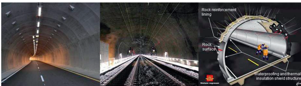
Figure 2. Recently constructed tunnel lining systems with drainage and thermal insulation shield structures as shown in fig 1. Left: Concrete segment shield structure for a highway tunnel. Middle: PE-foam shield structure in a high speed rail tunnel. Right: 3D image of the concrete segment and PE foam lining system highway tunnels (left and middle photos: Ådne Homleid/Byggeindustrien).
