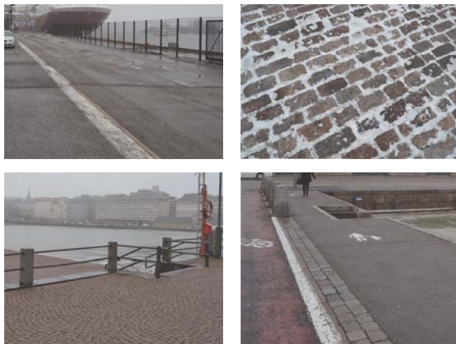
Ground materials at the old Harbour
