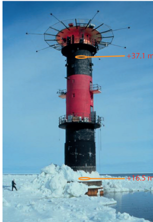
Figure 5. The Nordströmsgrund lighthouse: a) picture of the concrete structure in ice-infested water; b) force panels mounted to the outer face.
