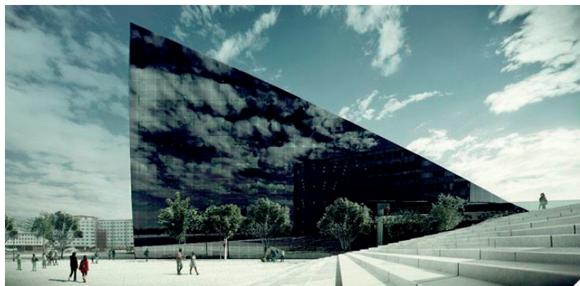
Figure 3: Powerhouse #1 at Brattøra port, Trondheim (Photo: www.powerhouse.no )
