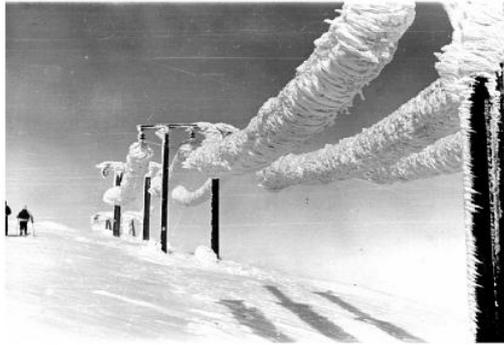
**Figure 1.1:** Rime icing on an electric powerline in Norway in April 1961.<sup>[3]</sup>
