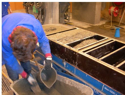
Figure 17: Casting of standard beams
