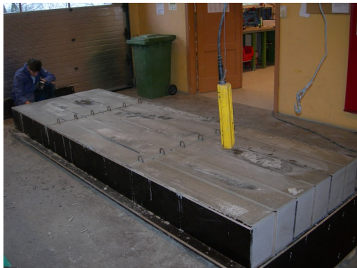
(a) Removing the formwork
