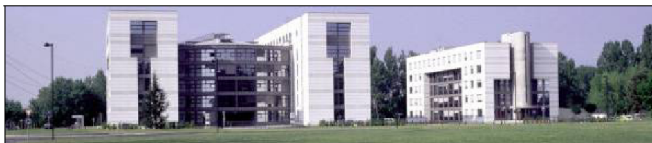
Figure 1. Building 40 and 39 on the Meyrin-site of CERN.
