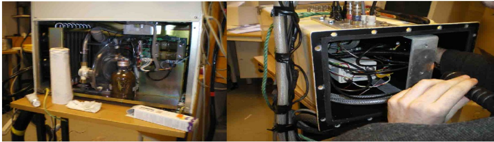
Figure 48: Fixing lidar system
