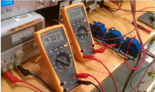
Figure 8.4.3.15: Multimeters for measuring inverter DC side voltage and current
