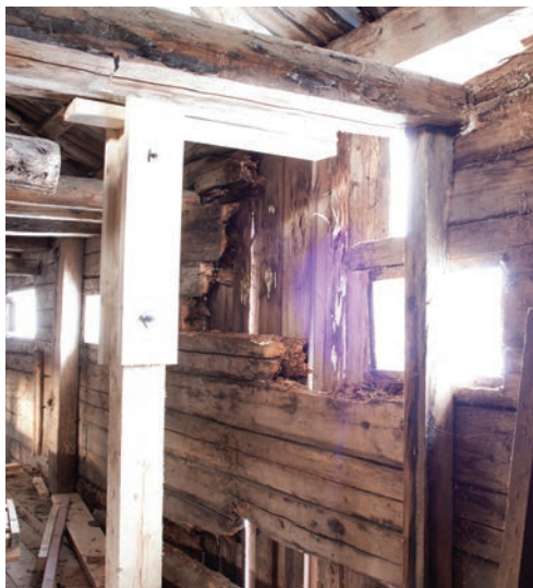
Hull i laft, 2. etg.
