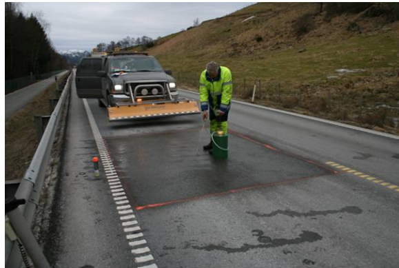
Figure 7 Dampening of a road section before use of the SOBO-20
