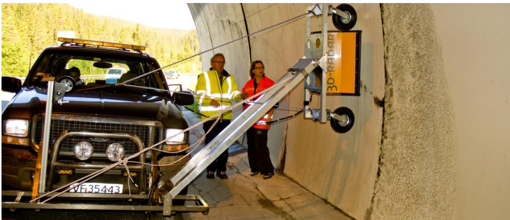
Figure 4 Vehicle bracket with arm mounted to allow surveying tunnel walls
