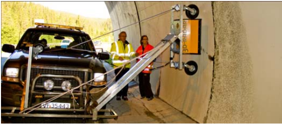
Figure 4. Vehicle bracket with arm mounted to allow surveying tunnel walls.
