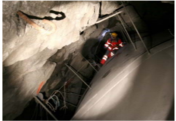
Figure 3. Space between the concrete vault and the rock surface
