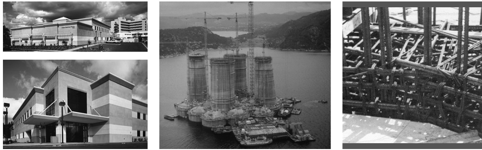
Figure 1.1: Concrete has become the most commonly used structural material used in modern civilizations. To the left is a typical concrete structure, while center demonstrates a construction of oil-platform, made of concrete. To the right: The flow of concrete inside a formwork is often made more difficult by the presence of congested reinforcement.
