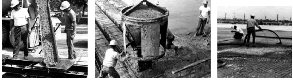
Figure 3.2: Different types of casting of the fresh concrete [24]. Here it is the dynamic yield value \tau_o that is more responsible for stopping the flowing concrete inside the formwork.
