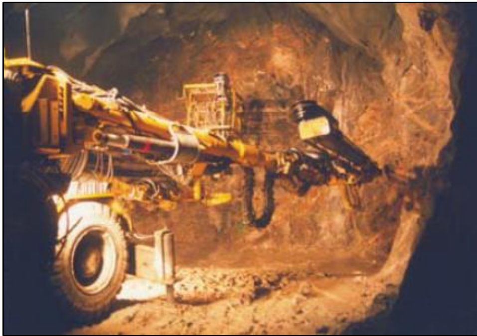
Figure 3-6: D&B excavation at the tunnel face (Nilsen, 2012).
